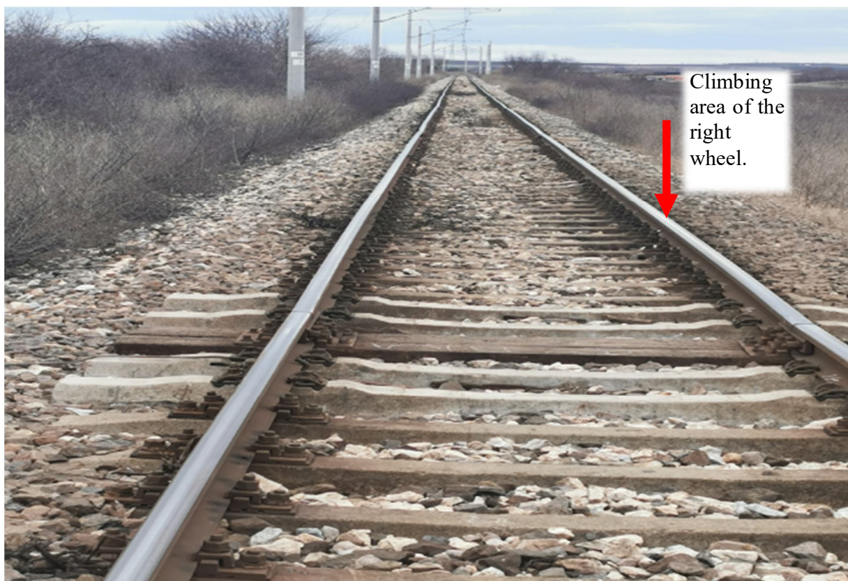
Fig. 1.2. The area of derailment of wagon № 21802475039-8 of IDFT № 46660
